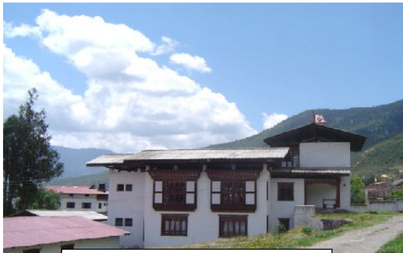
The Administration Block
